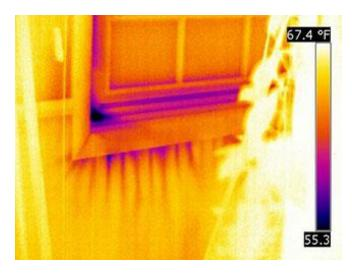
Cold air infiltrating at window casing trim and door threshold (below). *Invisible to the naked eye.*
