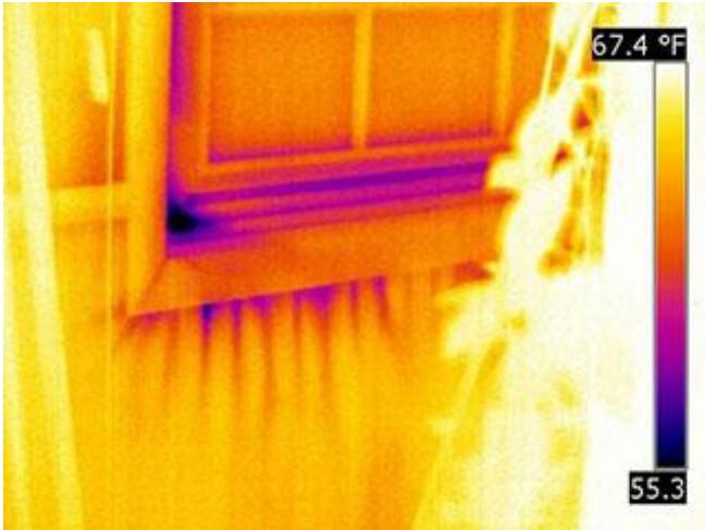
Cold air infiltrating at window casing trim and door threshold (below). *Invisible to the naked eye.*
