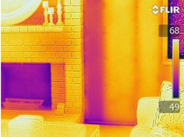
Missing and displaced insulation. *Invisible to the naked eye.*
